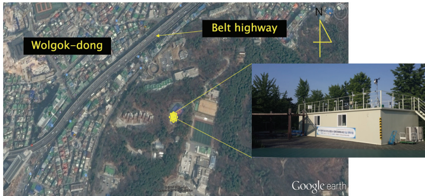
Fig. 1. Ground-base urban monitoring station at KIST (NIER, 2015).
